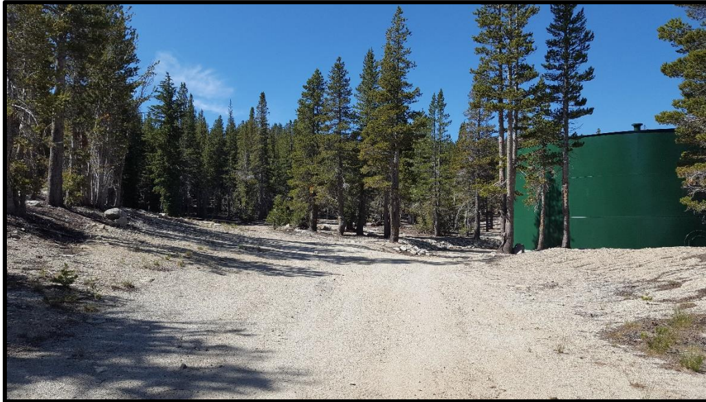
View to the south west toward proposed tank location, behind existing tank.
