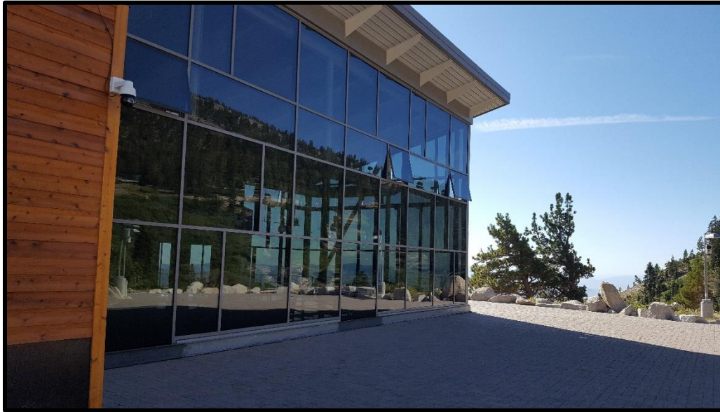
View of existing Winters Creek Lodge and patio to the southeast.
