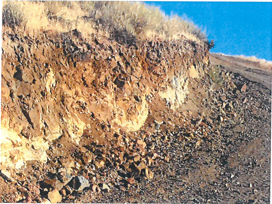
Close-up of cut slope on new driveway
