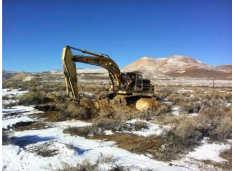
Test Pit Exploration
