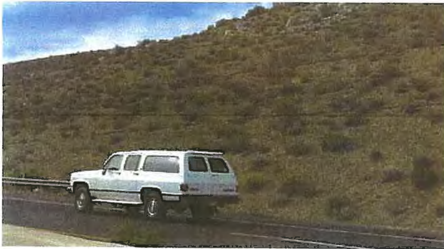
Naturalized rock cuts and grading that blend with the surrounding topography are preferred. Mass grading of slopes is visually unappealing and leads to vegetation management issues.
