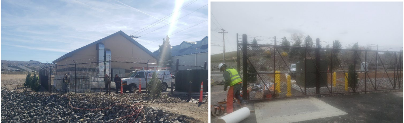
Examples of proposed 8 foot tall chain link fence with barbed wire top.
