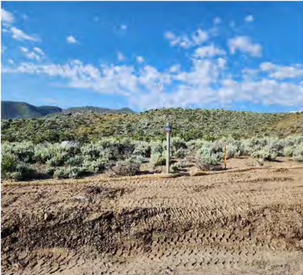
Photo 1: Looking South at Fiber Optic Cable Marker
