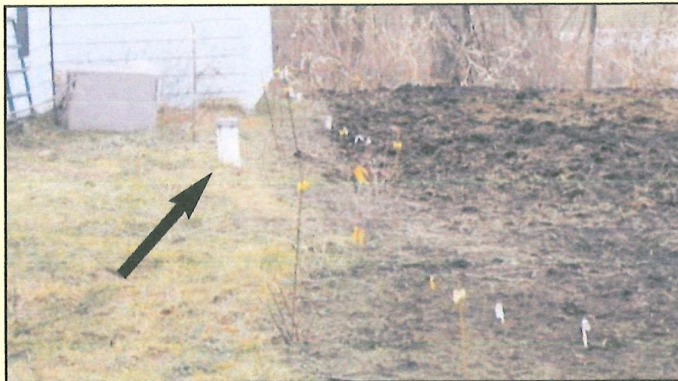
Figure 1. Horse lot within the 50-foot recommended isolation distance from well.
