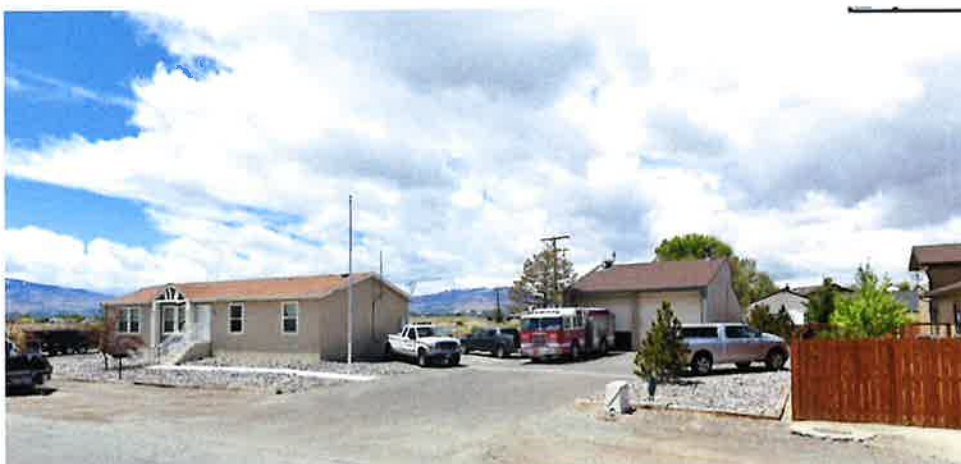
Existing Fire Station #37
