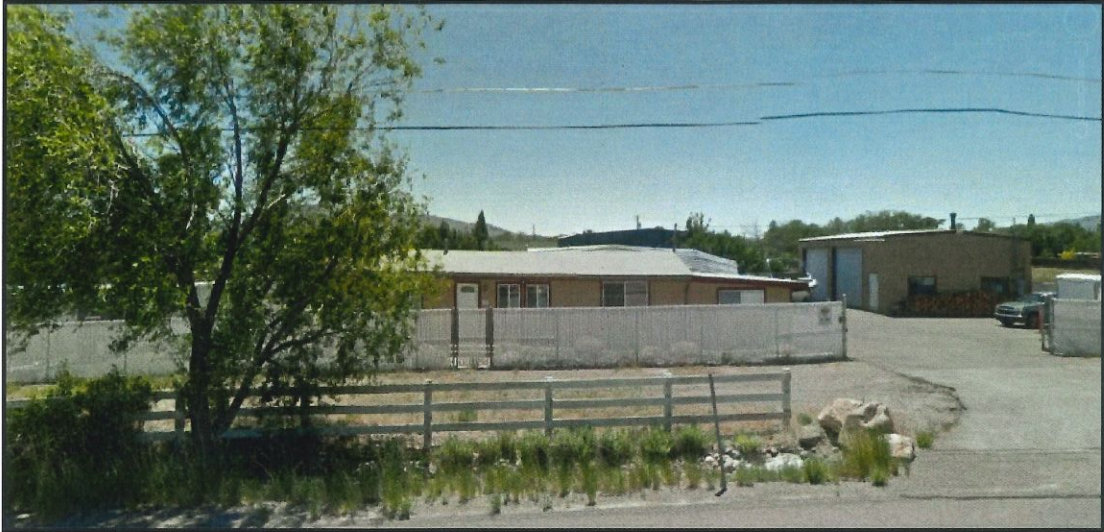
Photo 3: Development directly Northeast, Adjoining the Curtis & Sons Parcel
