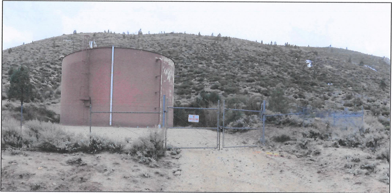
Figure 2 – Existing Conditions (Site Photo Looking South from Access Road)
