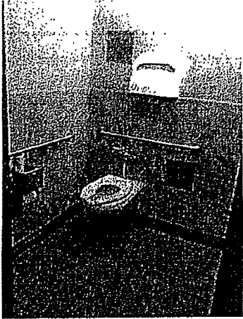
Prim Library ADA Accessible (no signs)
