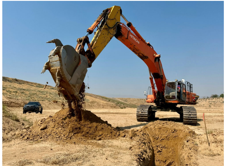
Test Pit Exploration
