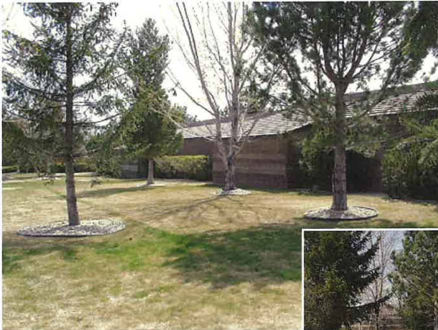
Photo A-3: Desirable Design Characteristics for Personal Storage Facilities
