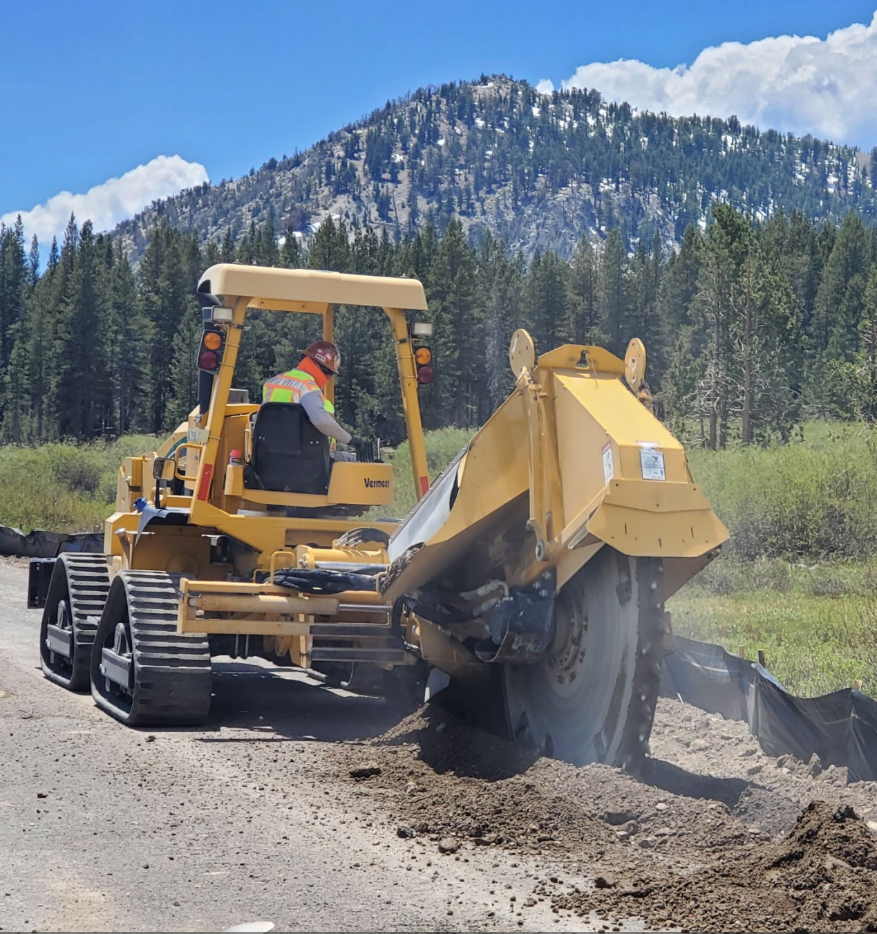
Rock saw used for ITS conduit installation
